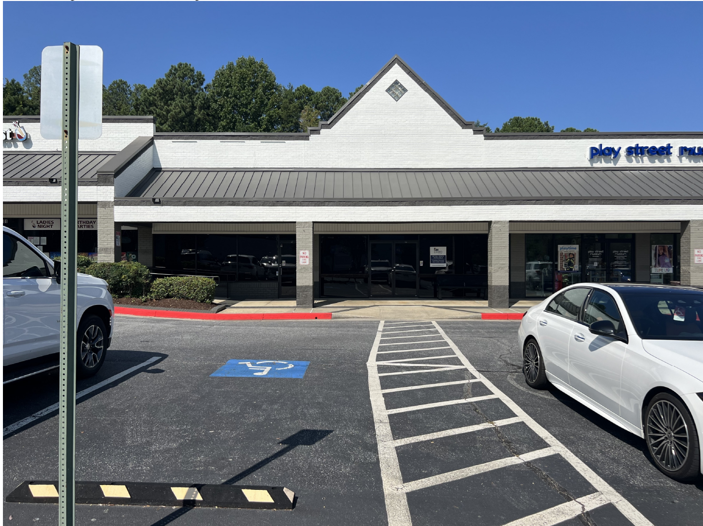
Existing Conditions of Building
