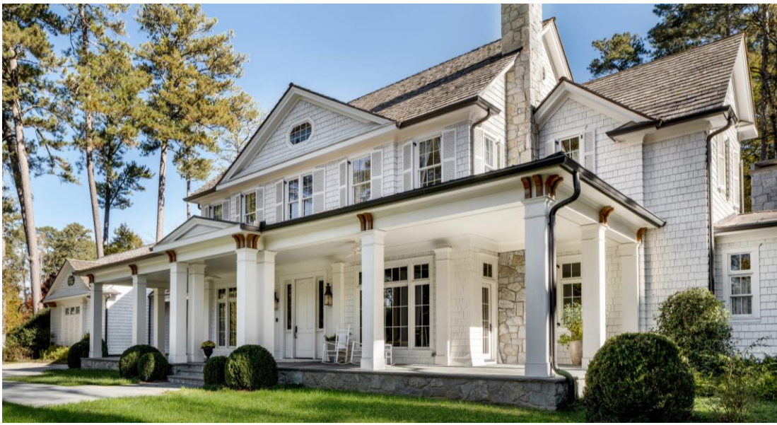
SQUARE COLUMNS, CEDAR SHINGLES & FRONT PORCH
