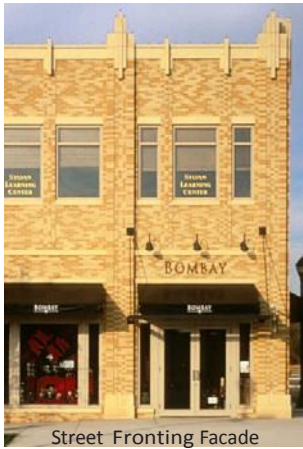
Street Fronting Facade
