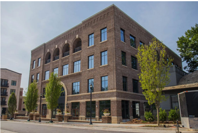
OFFICE/LABORATORY DEVELOPMENT PRECEDENT: DATA SCAN BUILDING, ALPHARETTA TOWN CENTER
