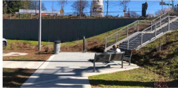
example of entrance plaza with exposed aggregate conc. finish
