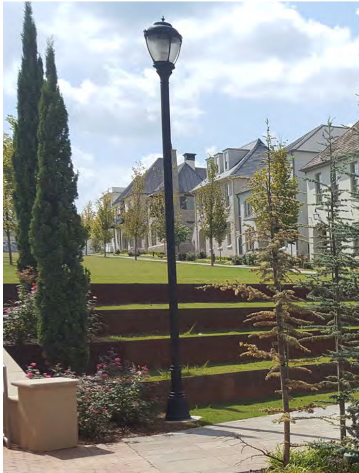
PEDESTRIAN LIGHT FIXTURE: GA POWER - GLANVILLE SERIES CITY OF ALPHARETTA STANDARD
