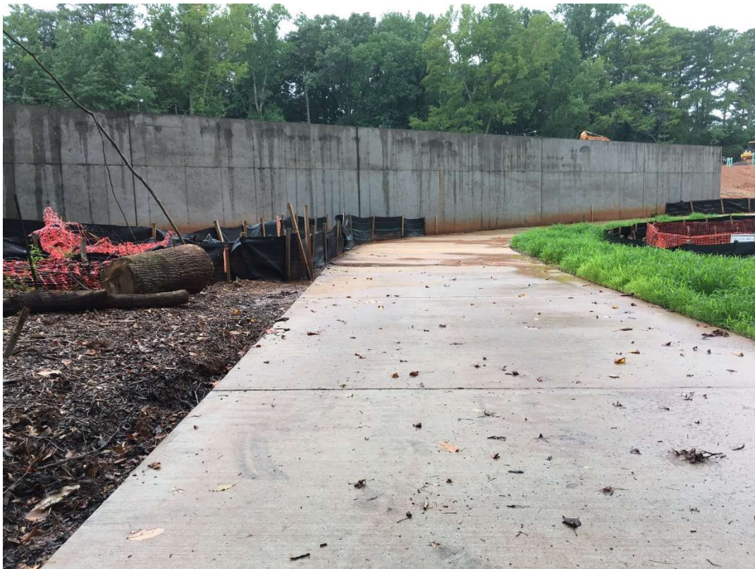
Photo 2. Detention pond wall looking west from Alpha Loop trail.
