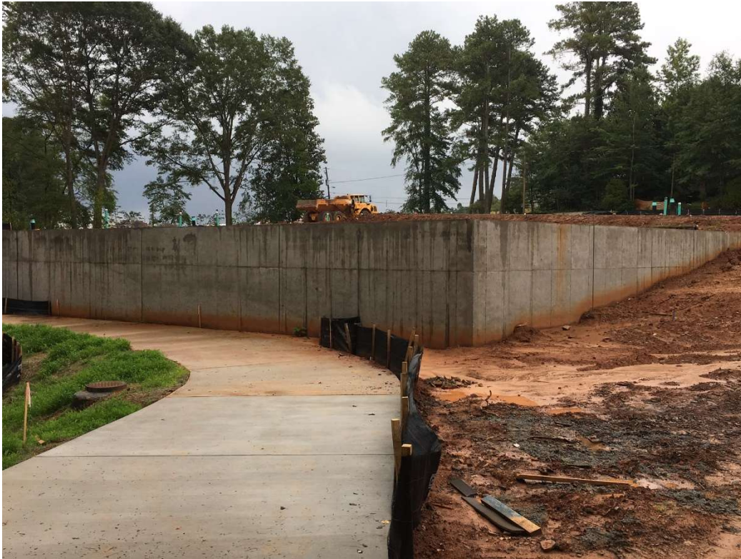
Photo 1. Detention Pond Wall looking east from Alpha Loop trail.
