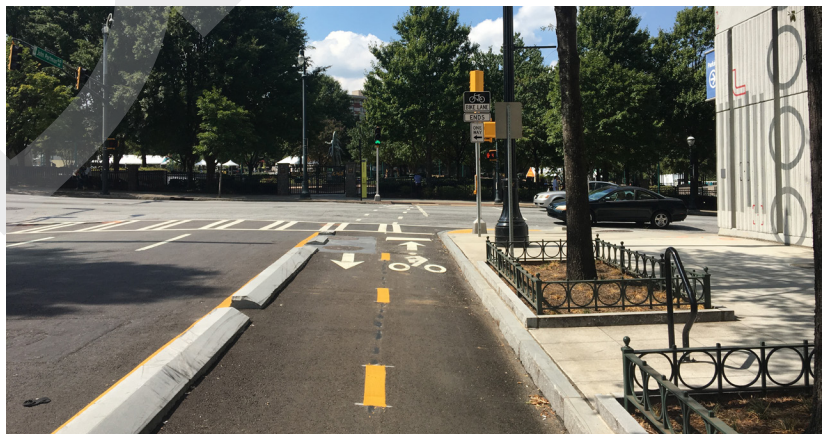
PROTECTED TWO-WAY CYCLE TRACK John Portman Boulevard, Atlanta, GA
