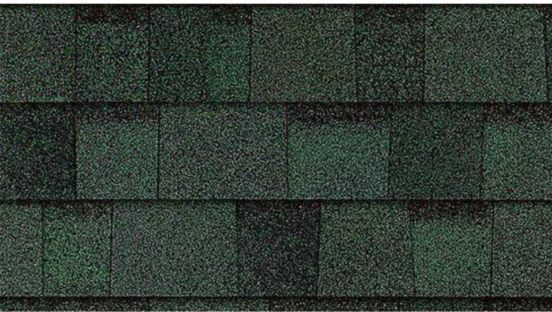
EXISTING GREEN ASPHALT SHINGLE ROOF
