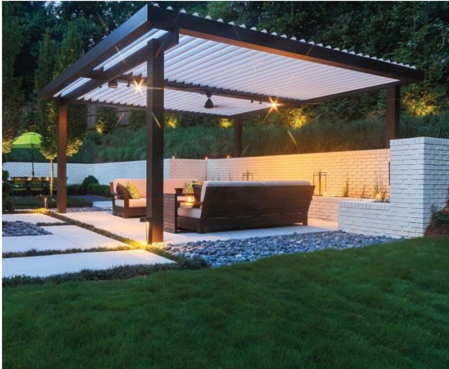
OPERABLE LOUVER ROTATES TO VARY THE AMOUNT OF ENCLOSURE.
