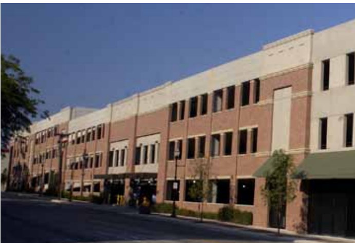
Parking Garage concealed behind decorative facade
