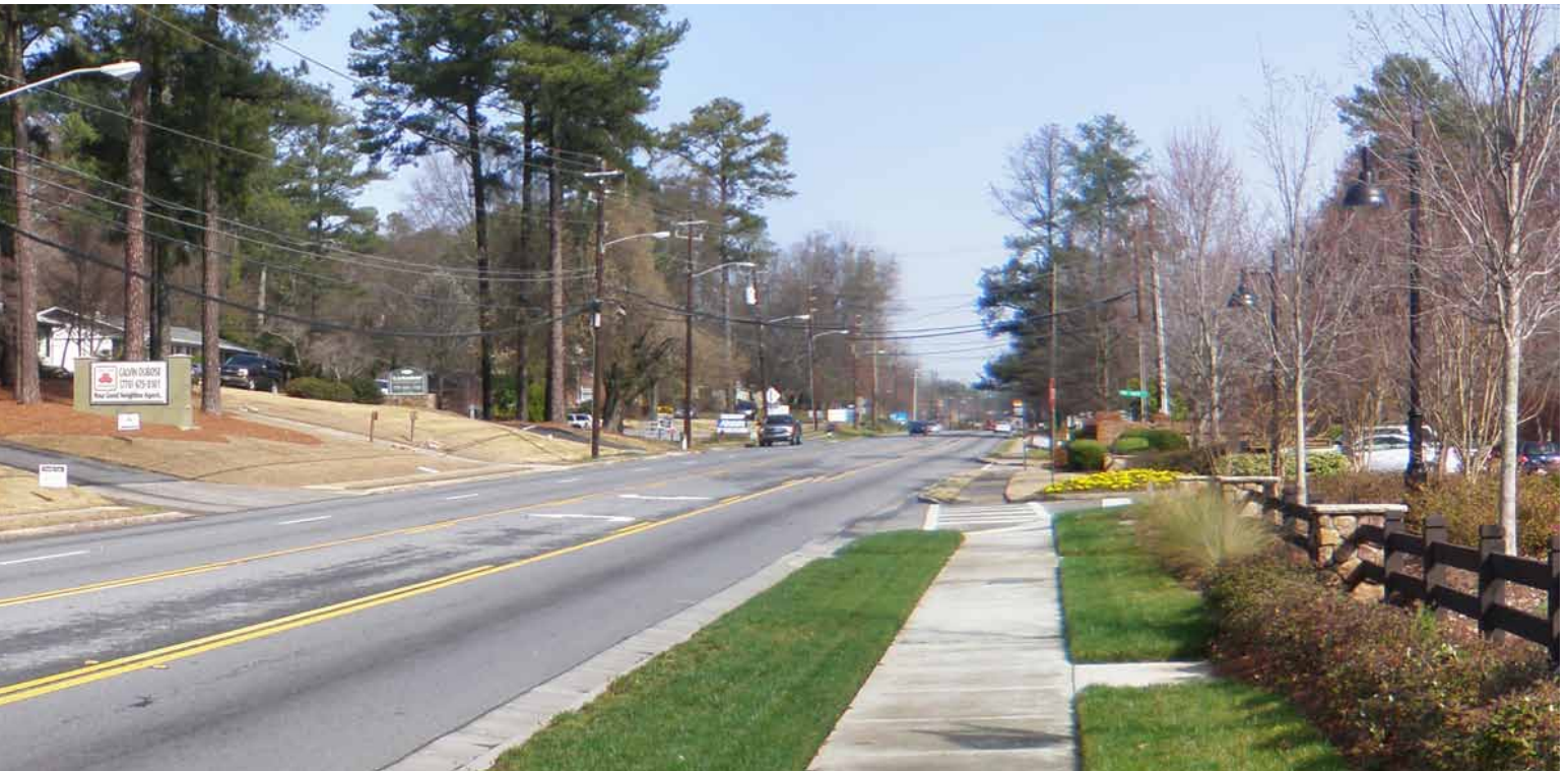
BEFORE: Highway 9 north of Mayfield Road, looking north
