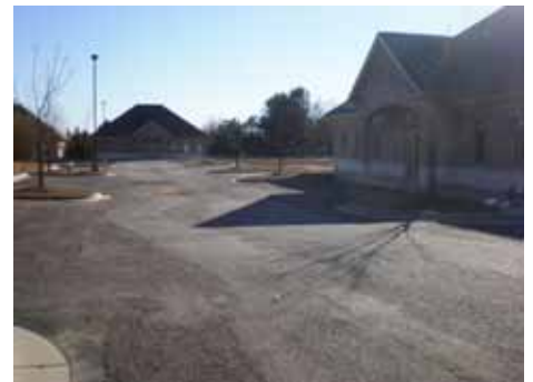
Unoccupied Office Development
