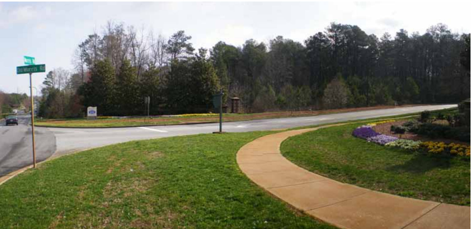
BEFORE: Intersection of Morris Road and Old Morris road looking north
