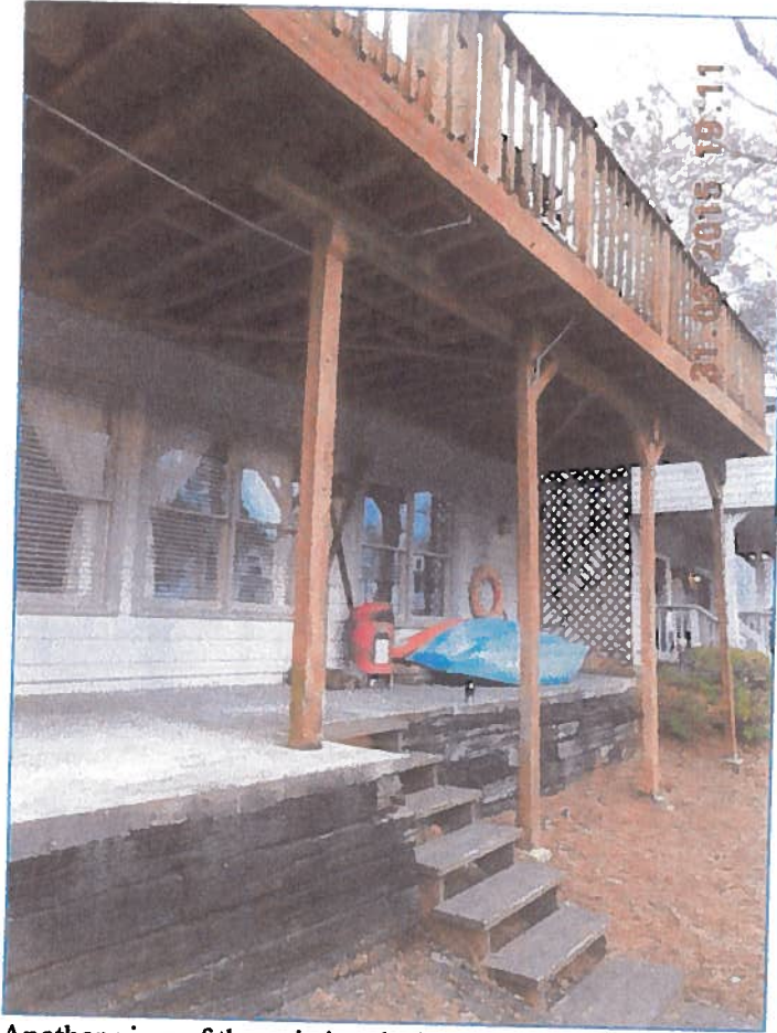
Another view of the existing deck, retaining wall and patio.
