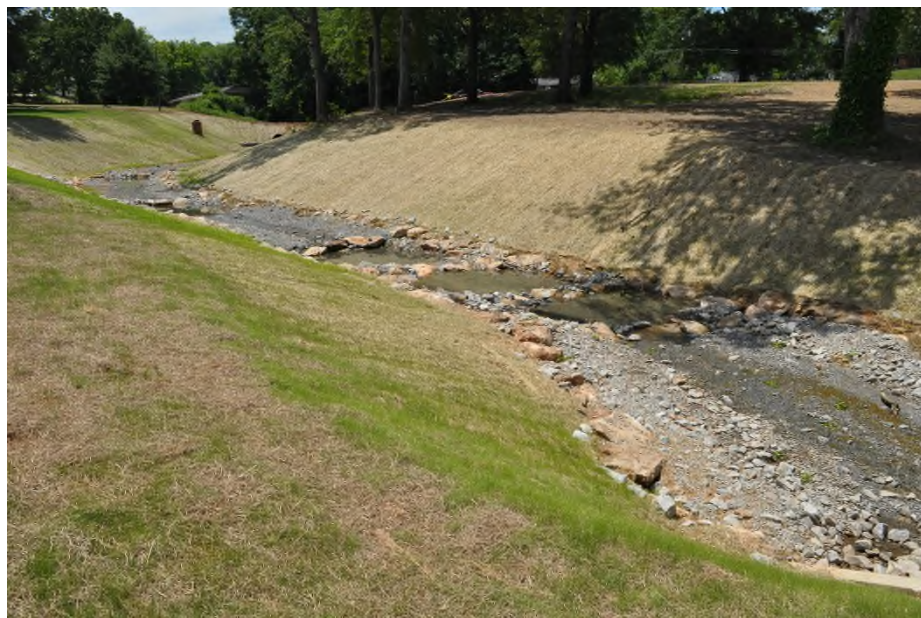
Kelsey Avenue Stream Restoration in Griffin, GA (Tetra Tech provided design, permitting and construction management for 960' of restoration)
