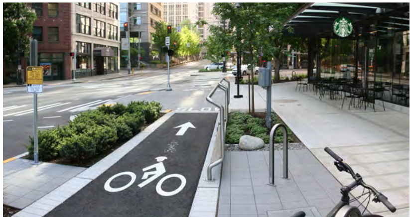
PROTECTED/ELEVATED ONE-WAY CYCLE TRACK 7th Avenue, Seattle, WA
