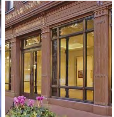
Examples of storefront that are composed of well-proportioned and detailed pilasters, mullions, and cornice trim.
