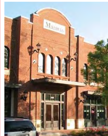
Larger glass areas are subdivided using elements of various width and amount of projection to provide a level of hierarchy within the opening.
