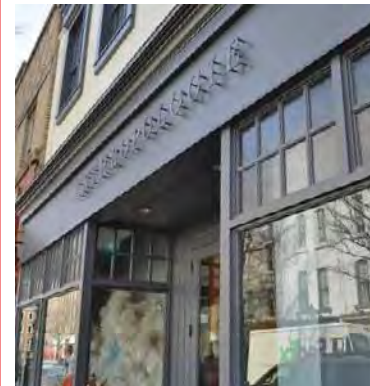
Larger glass areas are subdivided using elements of various width and amount of projection to provide a level of hierarchy within the opening.
