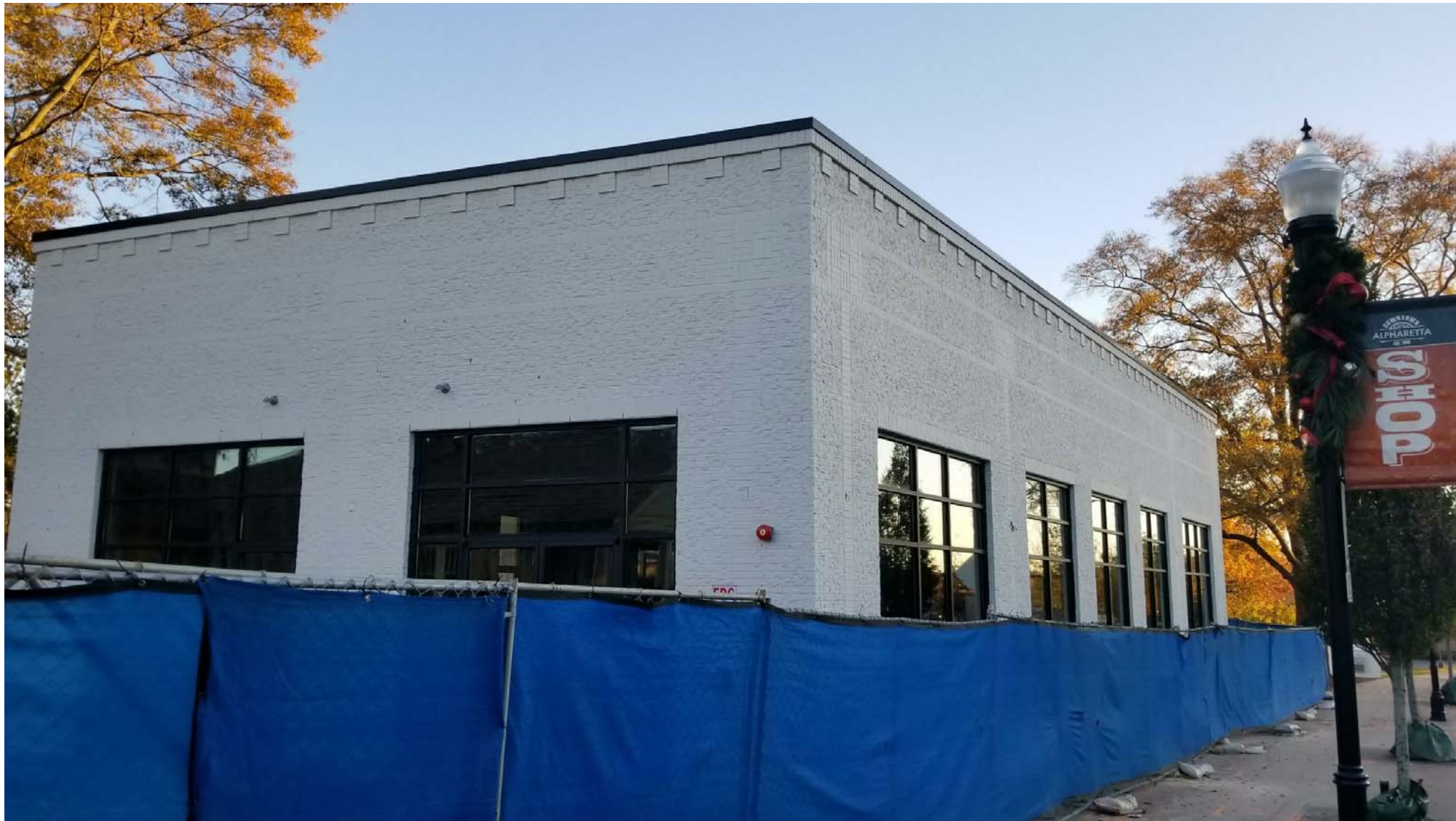
NEW CONSTRUCTION @ ALPHARETTA CITY CENTER LOC: 54 S MAIN STREET, ALPHARETTA
