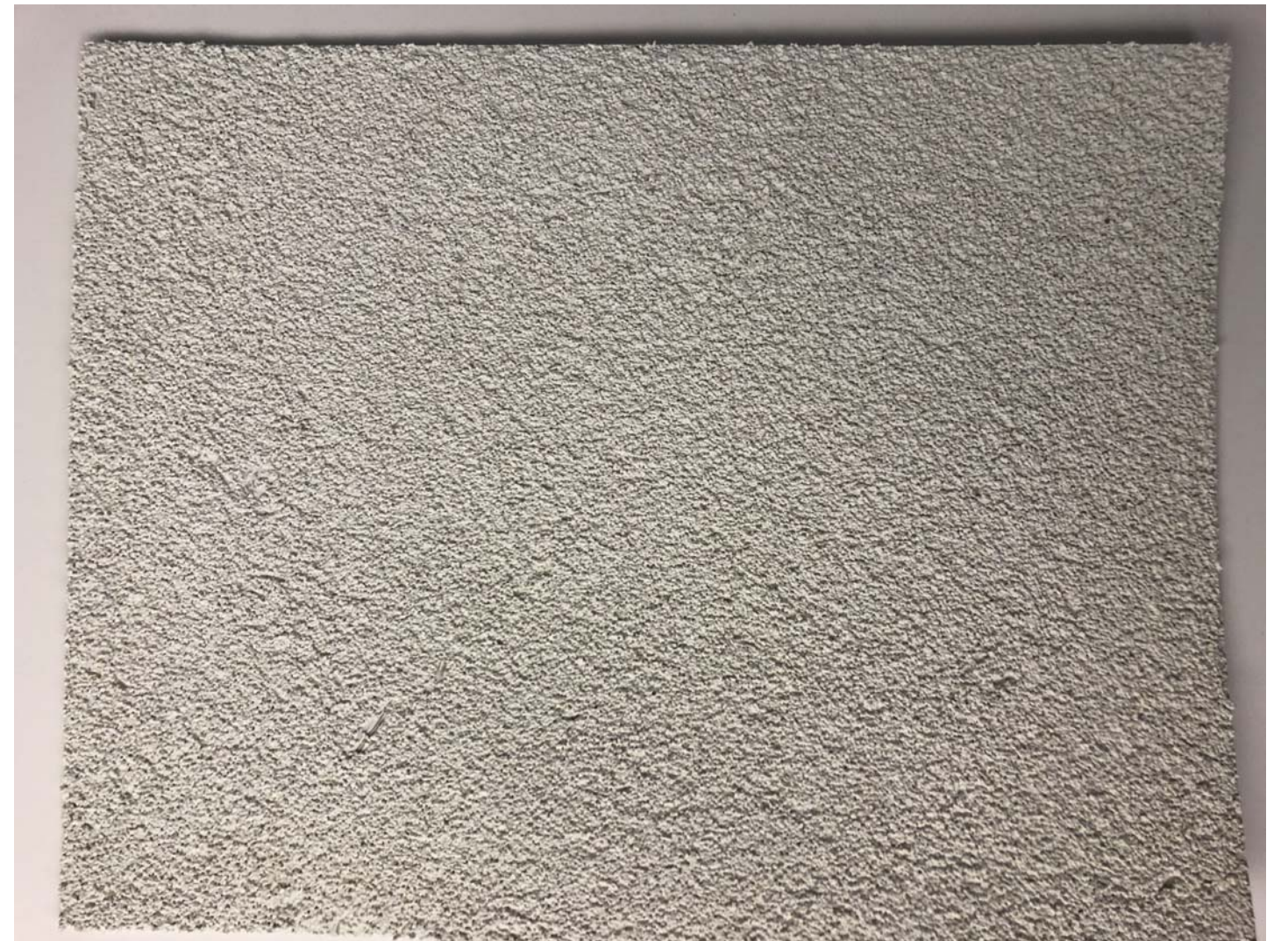
NEW STUCCO WALL, TO MATCH SENERGY ULTRA WHITE 330
