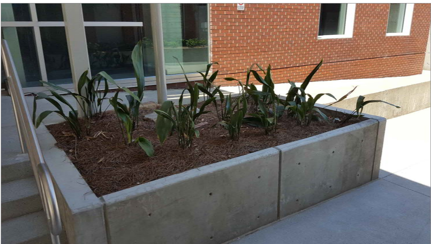
* CAST-IN-PLACE CONCRETE WALL W/ RUBBED FINISH (EXAMPLE)
