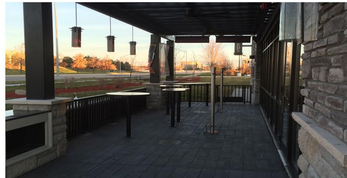
COVERED PATIO, WEST DES MOINES, IOWA
