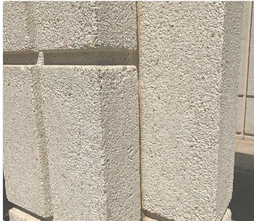
TEXTURE OF EXISTING BUILDING
