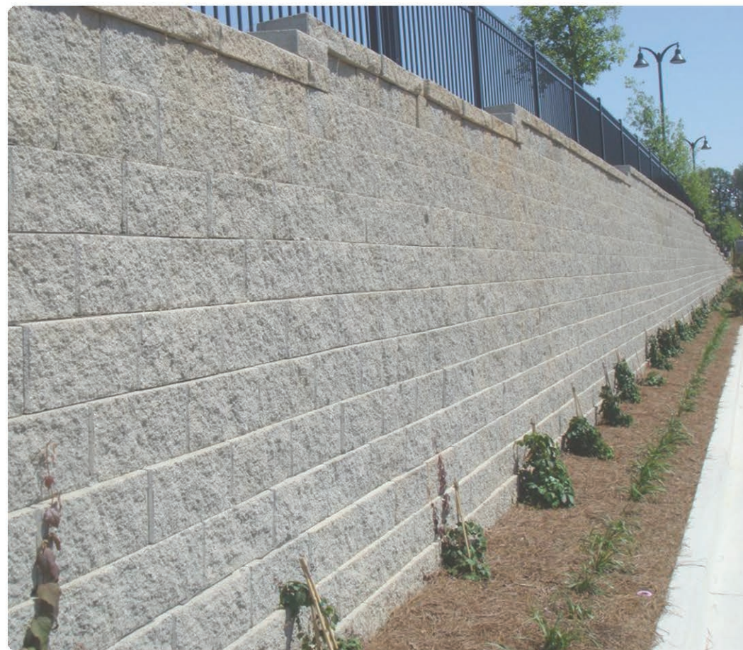
MODULAR BLOCK RETAINING WALL
