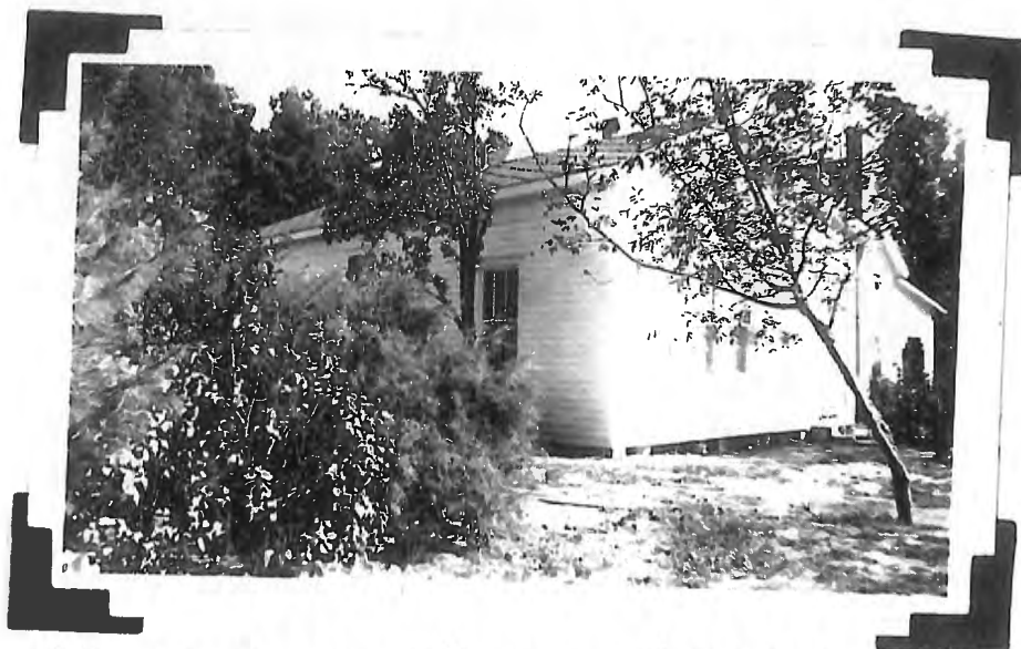
Close view of new addition.
