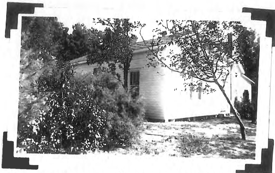
Close view of new addition.
