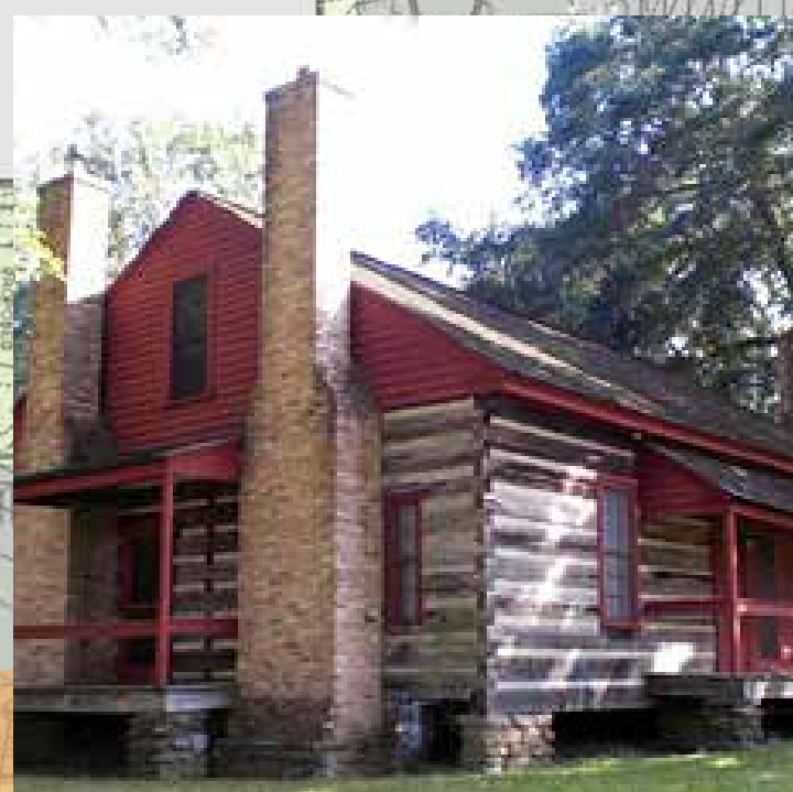
RECONSTRUCTION HISTORIC CABIN (COMMUNITY PROJECT)
