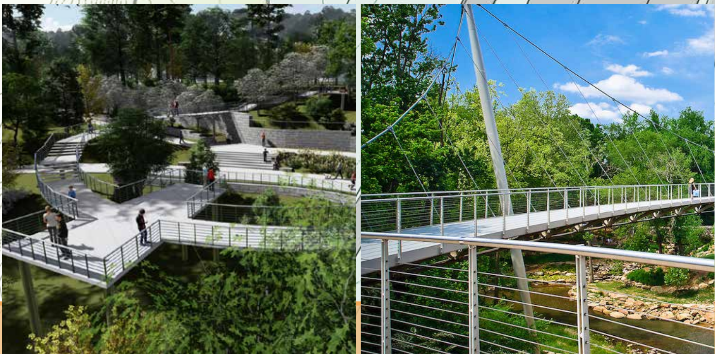
MAJOR ELEVATED STRUCTURE
