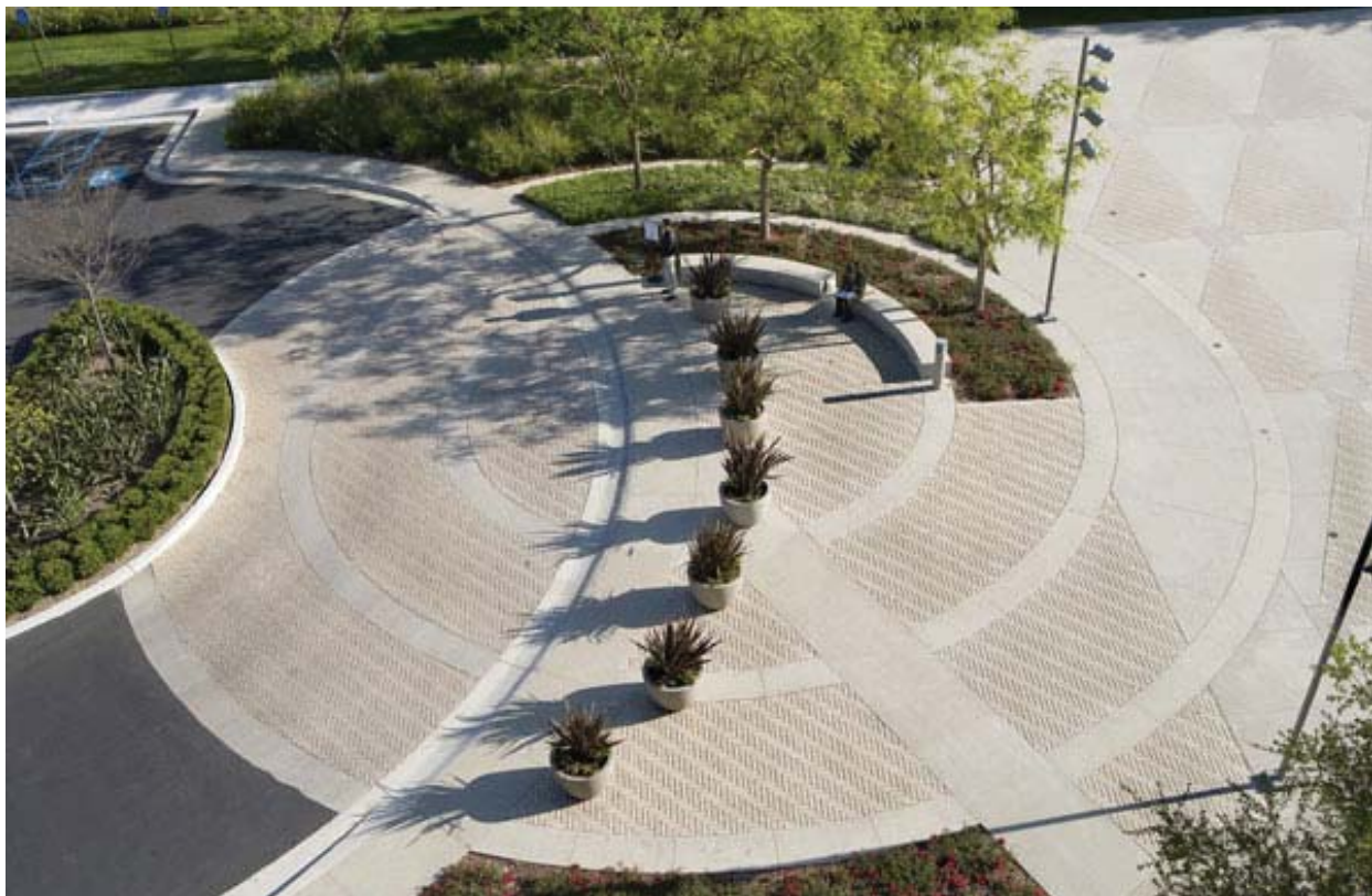
ENHANCED CONCRETE PAVEMENTS: EXAMPLE 1 INTEGRAL COLOR, DECORATIVE JOINTS, TEXTURED FINISH
