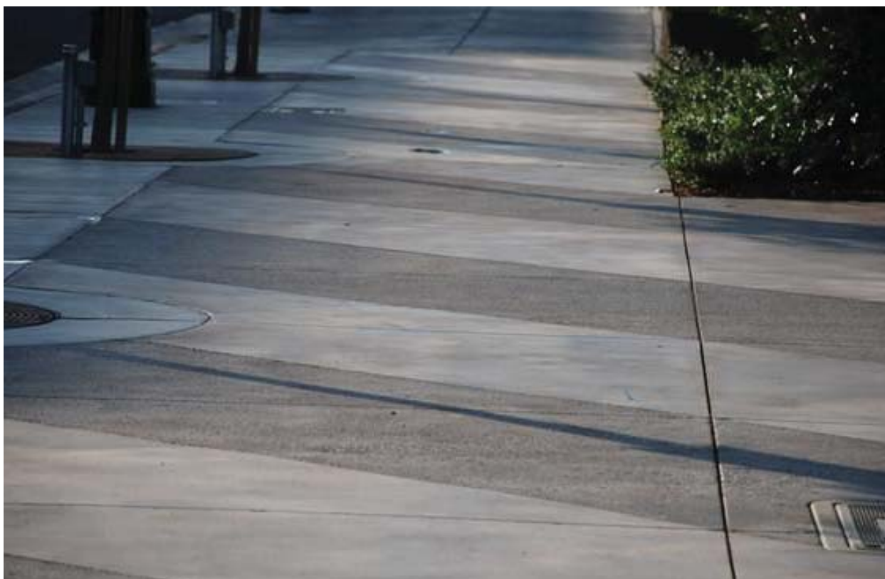
ENHANCED CONCRETE PAVEMENTS: EXAMPLE 2 INTEGRAL COLOR, DECORATIVE JOINTS, TEXTURED FINISH
