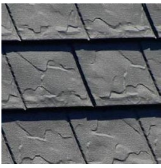
PORTICO ROOF TILE IRONSTONE SLATE
