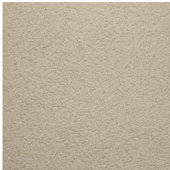
STUCCO (AT REAR FACADE) “FUNCTIONAL GRAY”
