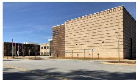
5. Northwest Corner, Gymnasium
