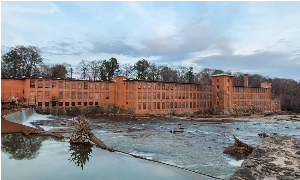
Porterdale Mill Lofts - Covington, GA
