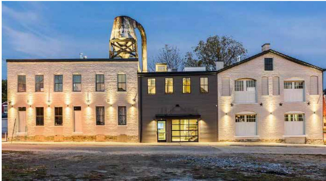
Hellman Lumber Building - Covington KY
