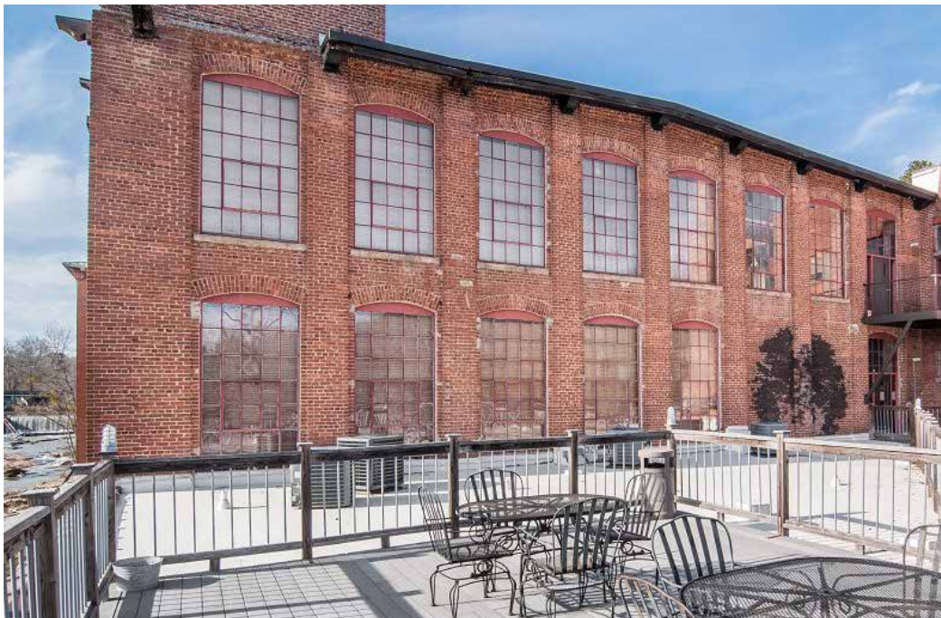
Porterdale Mill Lofts - Covington, GA
