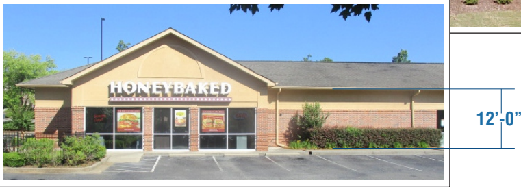
STOREFRONT (East) ELEVATION - Left end of bldg
