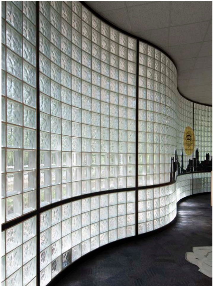
The piano shaped glass block wall is a key architectural feature of the Library. It provides sufficient diffused light but does not allow for visible connectivity or access between the inside and outside of the building.
