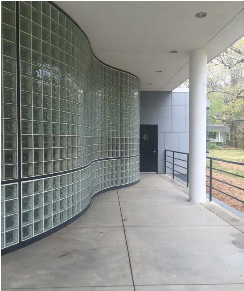
The piano shaped glass block wall is a key architectural feature of the Library. It provides sufficient diffused light but does not allow for visible connectivity or access between the inside and outside of the building.
