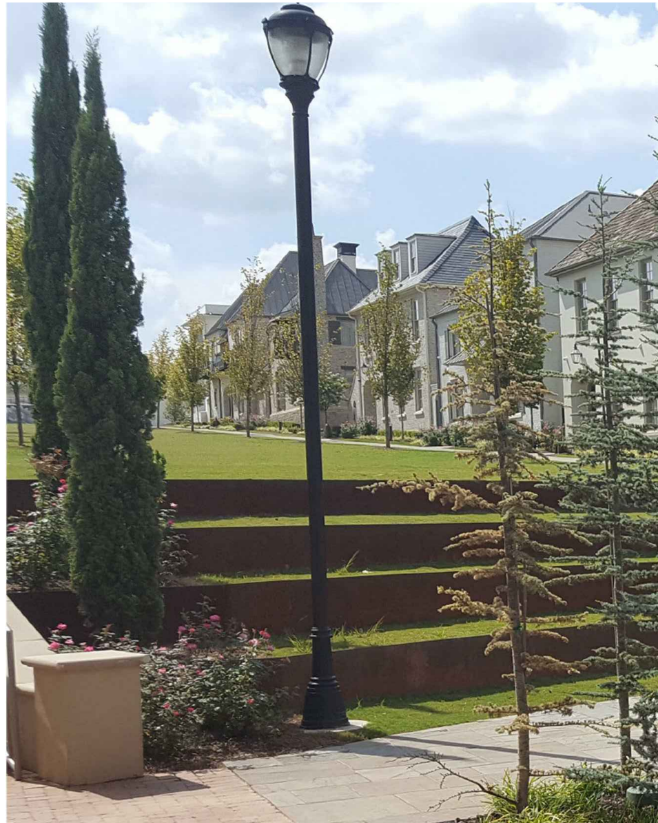
INFRASTRUCTURE PROJECT PEDESTRIAN LIGHT FIXTURE
