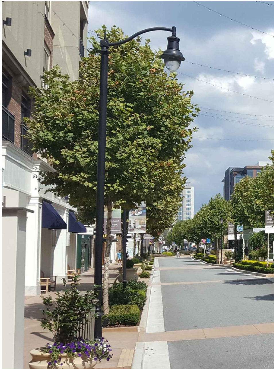
INFRASTRUCTURE PROJECT STREET LIGHT FIXTURE
