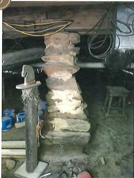
STONE PIERS AND MORTAR & TENON BEAMS AND JOISTS
