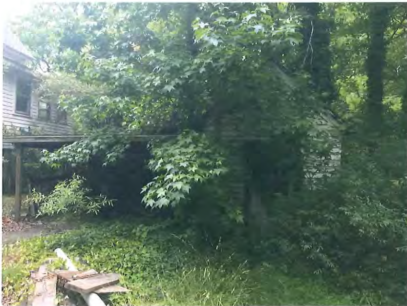
SINGLE PEN SHED - LIKELY ORIGINAL TO HOUSE
