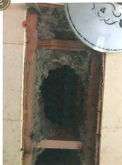
NOTE ORIGINAL TONGUE AND GROVE PAINTED PINE CEILING 5 FEET ABOVE ADDED CEILING.
