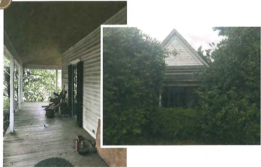
SIMPLIFIED VICTORIAN AND QUEEN ANNE ELEMENTS TYPICAL OF FOLK VICTORIAN STYLE POSTS (LEFT) AND GABLE (RIGHT)
