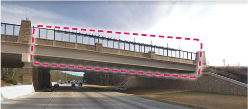
GA 400 VIEW: PARAPET WALLS, BEAMS (OUTSIDE AND CENTER)
