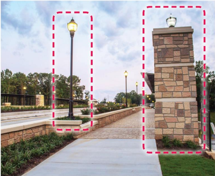
LARGE COLUMNS AND PEDESTRIAN LIGHTING
