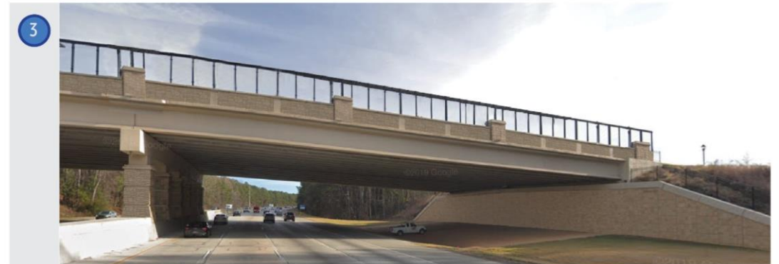
SMALL COLUMNS THROUGHOUT
