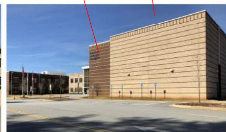
5. Northwest Corner, Gymnasium
