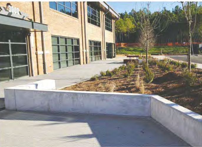
(PHOTO SHOWN FROM NORTHWINDS BUILDING 3000 PROJECT)
