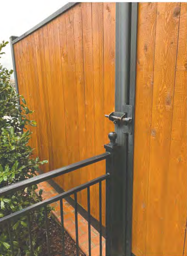
SCREEN/FENCE @ TRASH/TRANSFORMER/GENERATOR ENCLOSURE: CUSTOM SEGMENTED AND REMOVABLE FENCING & GATE - 8' HT. -BLACK STEEL FRAME W/ STAINED CEDAR INFILL
