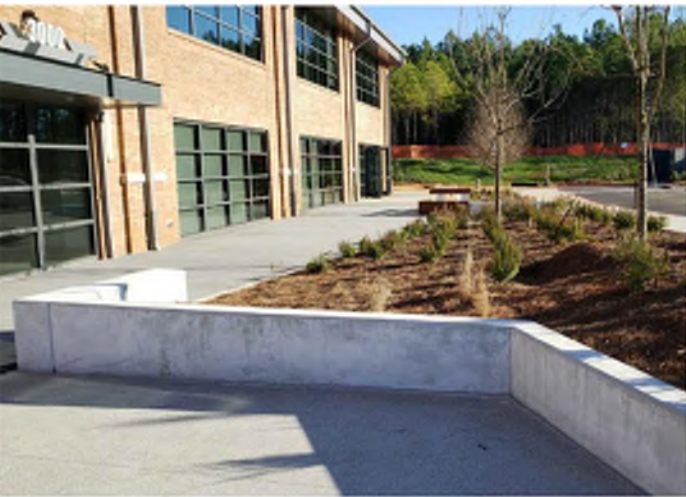
(PHOTO SHOWN FROM NORTHWINDS BUILDING 3000 PROJECT)
