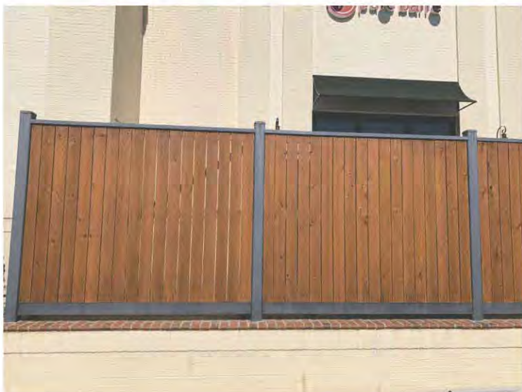
SCREEN/FENCE @ TRASH/TRANSFORMER/GENERATOR ENCLOSURE: CUSTOM SEGMENTED AND REMOVABLE FENCING & GATE - 8' HT. -BLACK STEEL FRAME W/ STAINED CEDAR INFILL
