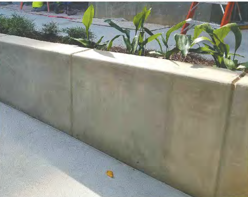
CAST-IN-PLACE CONCRETE RETAINING WALL RUBBED FINISH
