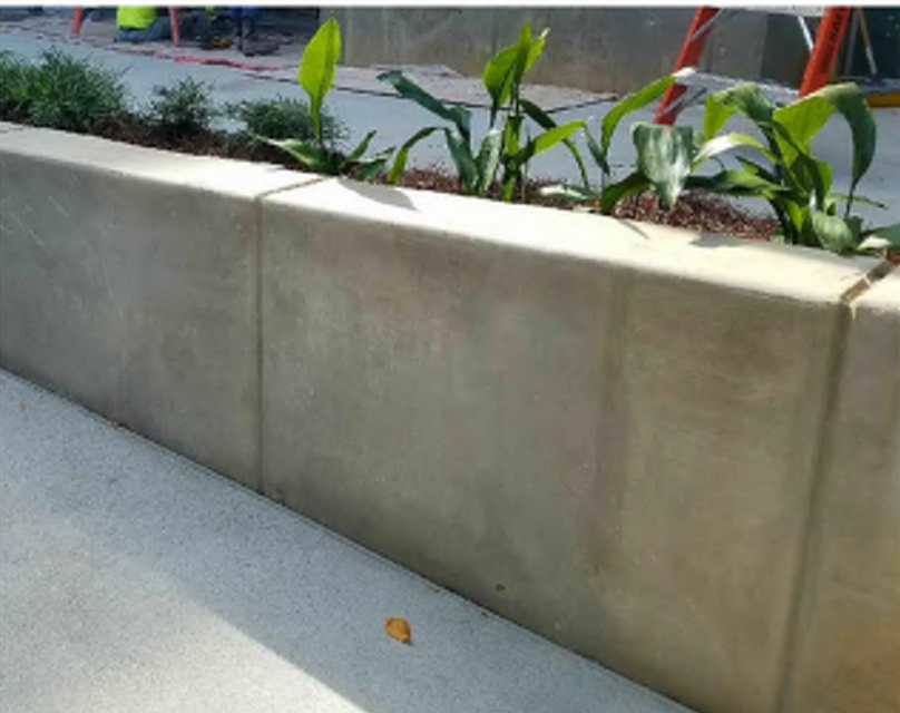
CAST-IN-PLACE CONCRETE RETAINING WALL RUBBED FINISH
