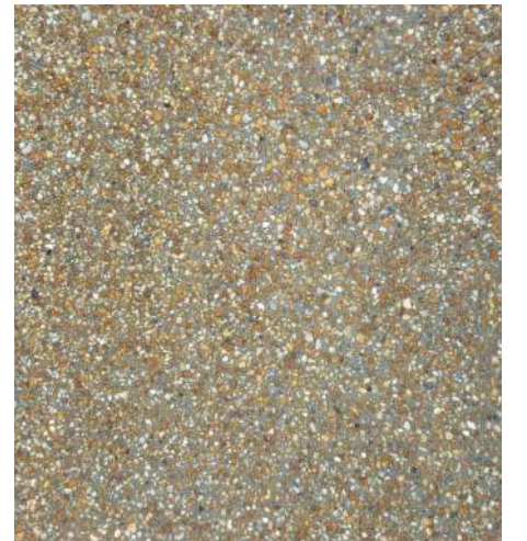
enhanced pedestrian concrete
