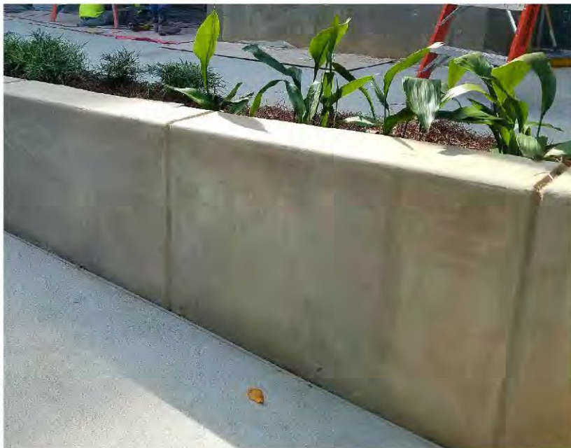
CAST-IN-PLACE CONCRETE RETAINING WALL RUBBED FINISH
