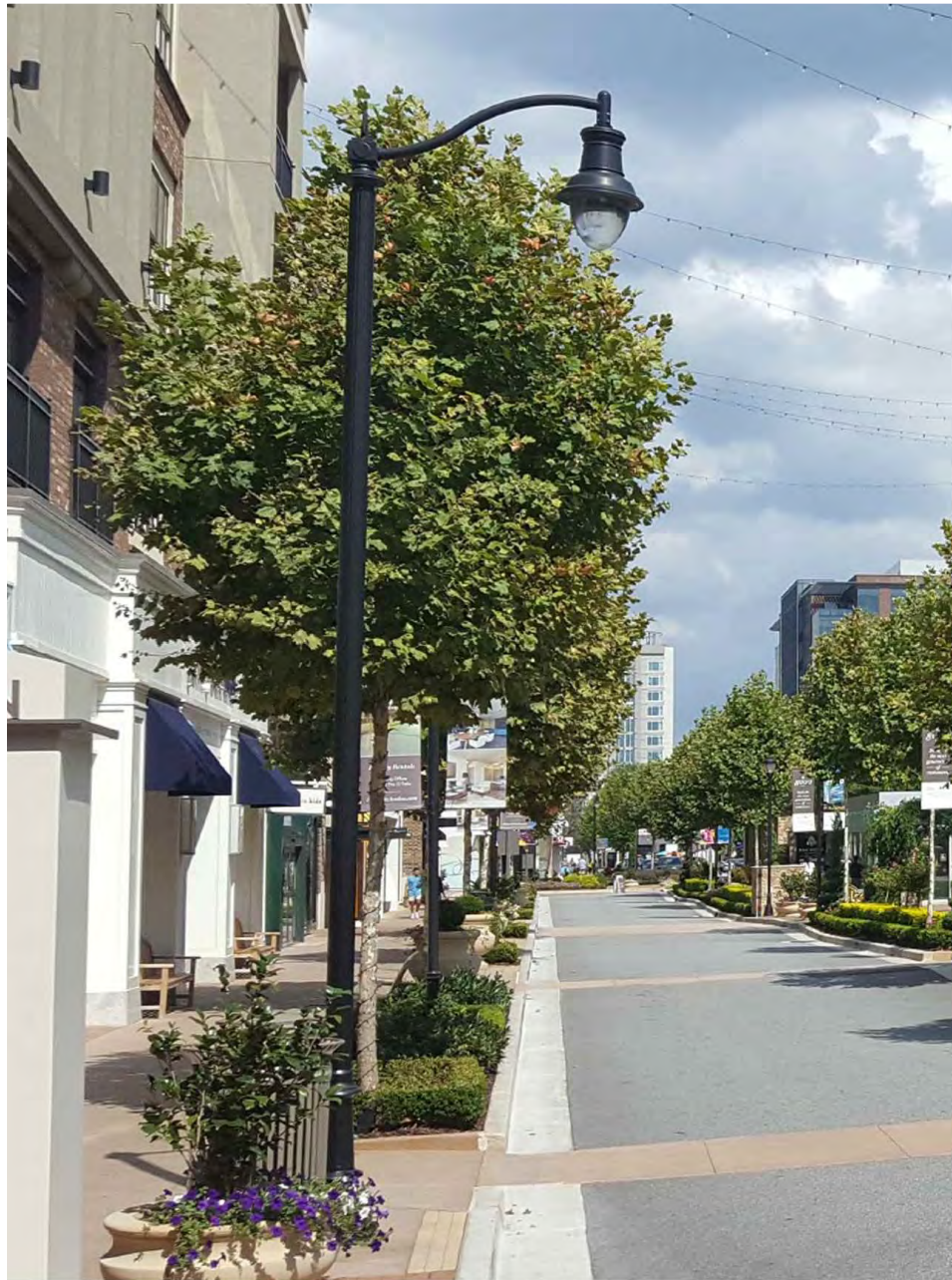
INFRASTRUCTURE PROJECT STREET LIGHT FIXTURE
