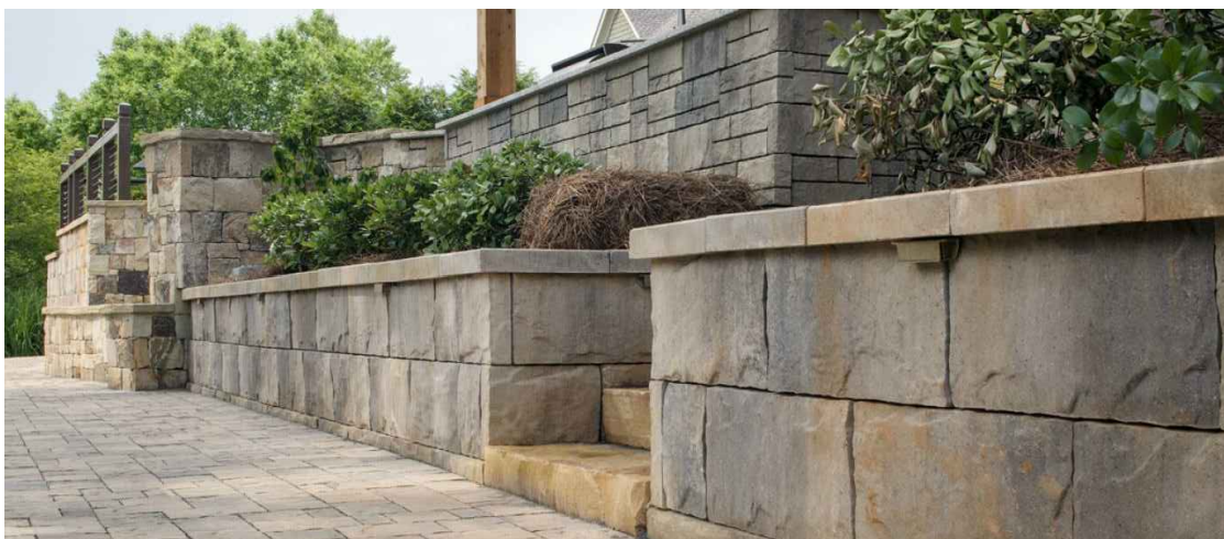
SEGMENTAL BLOCK RETAINING WALL (BELGARD: MEGA TANDEM STONE)
