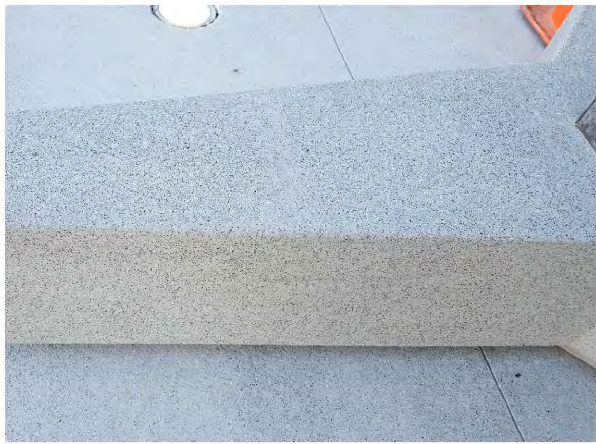
DECORATIVE CONCRETE SIDEWALK (INTEGRAL COLOR W/ BLACK BEAUTY SAND & LIGHT TOP CAST)
