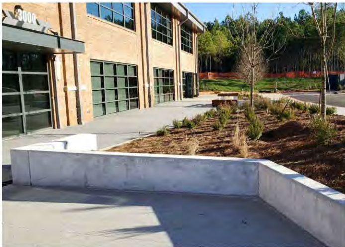
(PHOTO SHOWN FROM NORTHWINDS BUILDING 3000 PROJECT)
