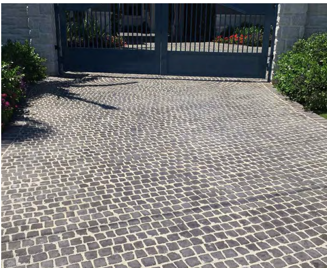
FAUX COBBLESTONE PAVEMENT (RIGGIBENE: COBBLESYSTEM - CHARCOAL)
