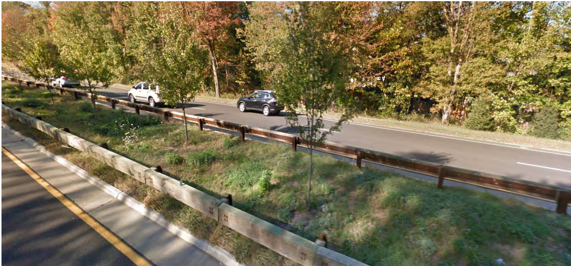
Steel-backed Timber Guardrail (CT-15 / Merritt Parkway, New Canaan, CT.)
