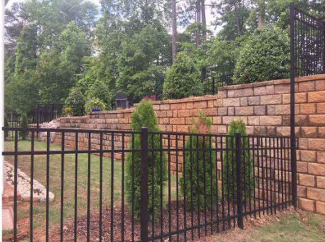
LOT #37 BACKYARD RETAINING WALL
