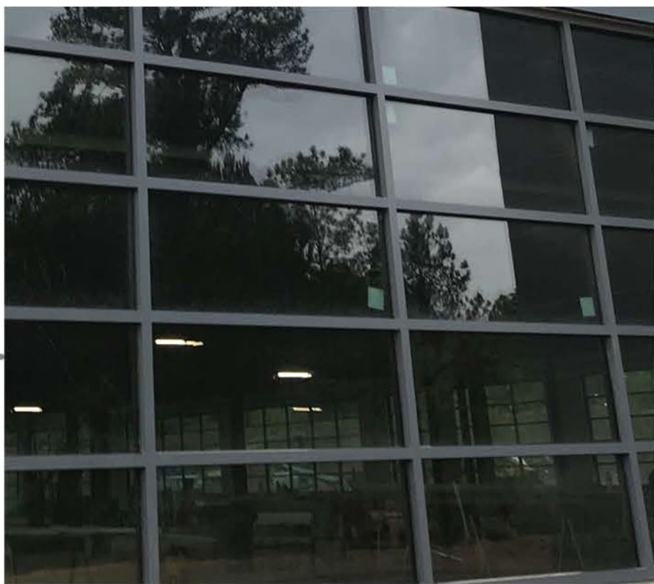
WINDOW WALL SYSTEM GLAZING: VIRACON VNE 19-63 ALUMINUM MULLION COLOR: CHARCOAL
