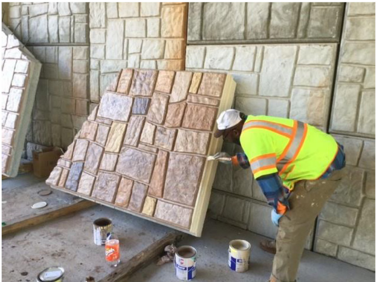
ENCORE PARKWAY BRIDGE WALL MOCKUP PHOTOS
