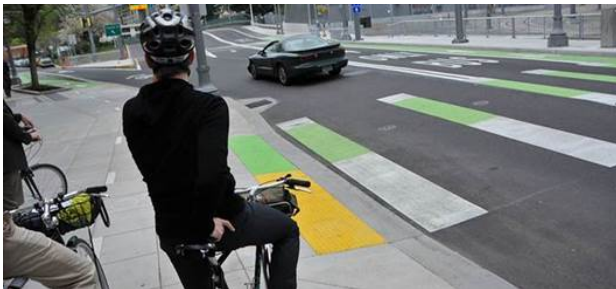
Figure 1: Split Bike/Ped Crossing Detectable Warning
