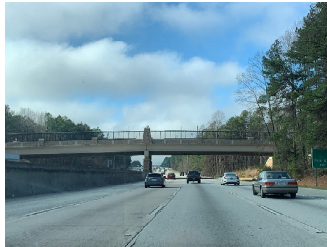
Georgia 400 southbound approaching Encore Parkway bridge
