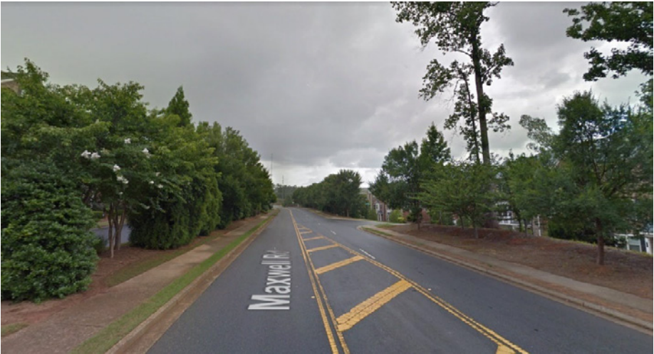
Maxwell Road south of Westside Parkway
