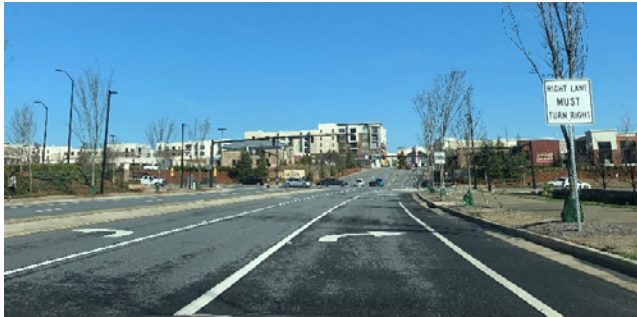
New multiuse path on North Winds Parkway approaching Avalon
