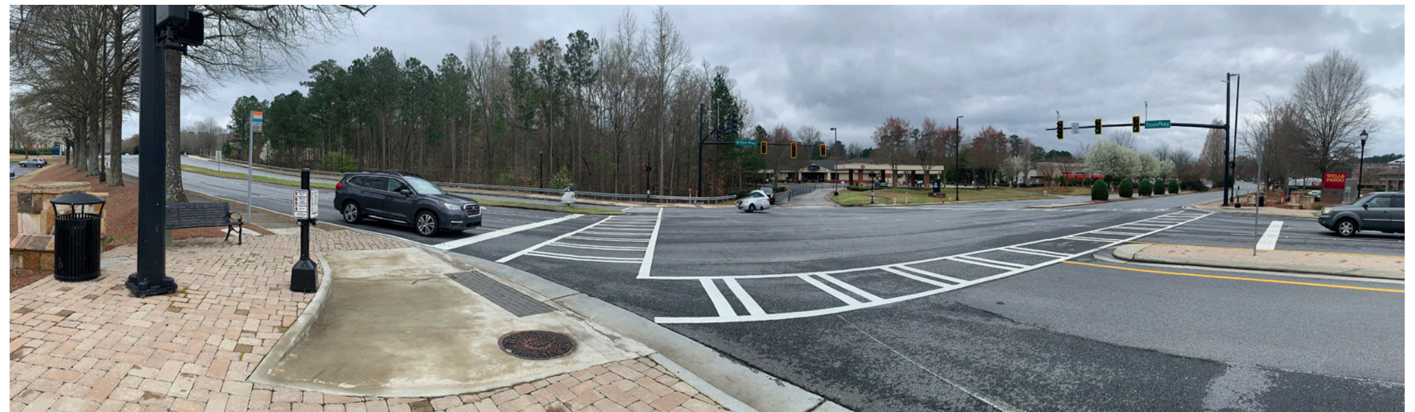
North Point Pkwy & Encore Pkwy (looking south)
