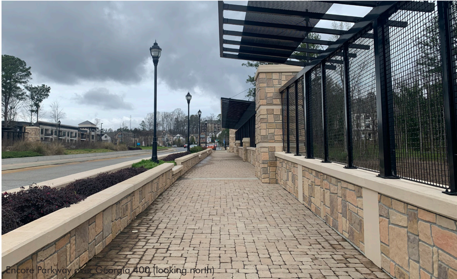
Haynes Bridge Road near Georgia 400 Southbound (looking south)
