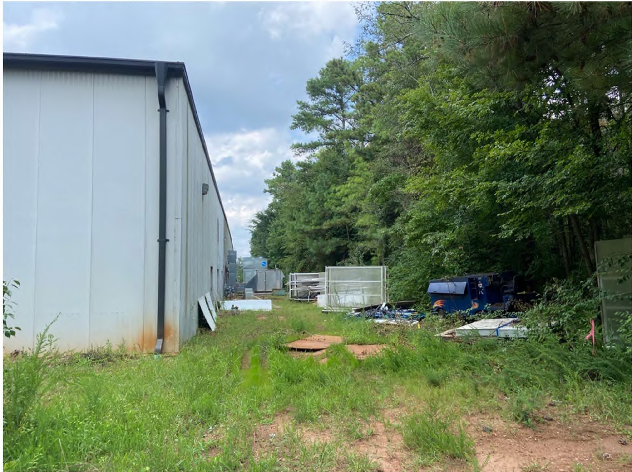
2. COOLER - REAR VIEW
