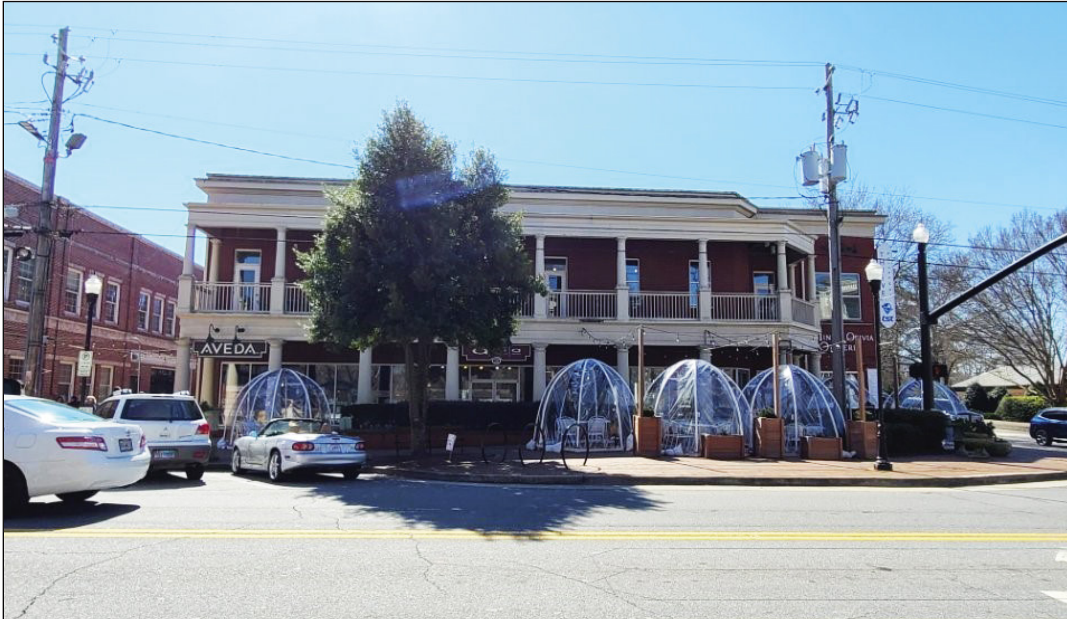
EXISTING BUILDING FACADE
