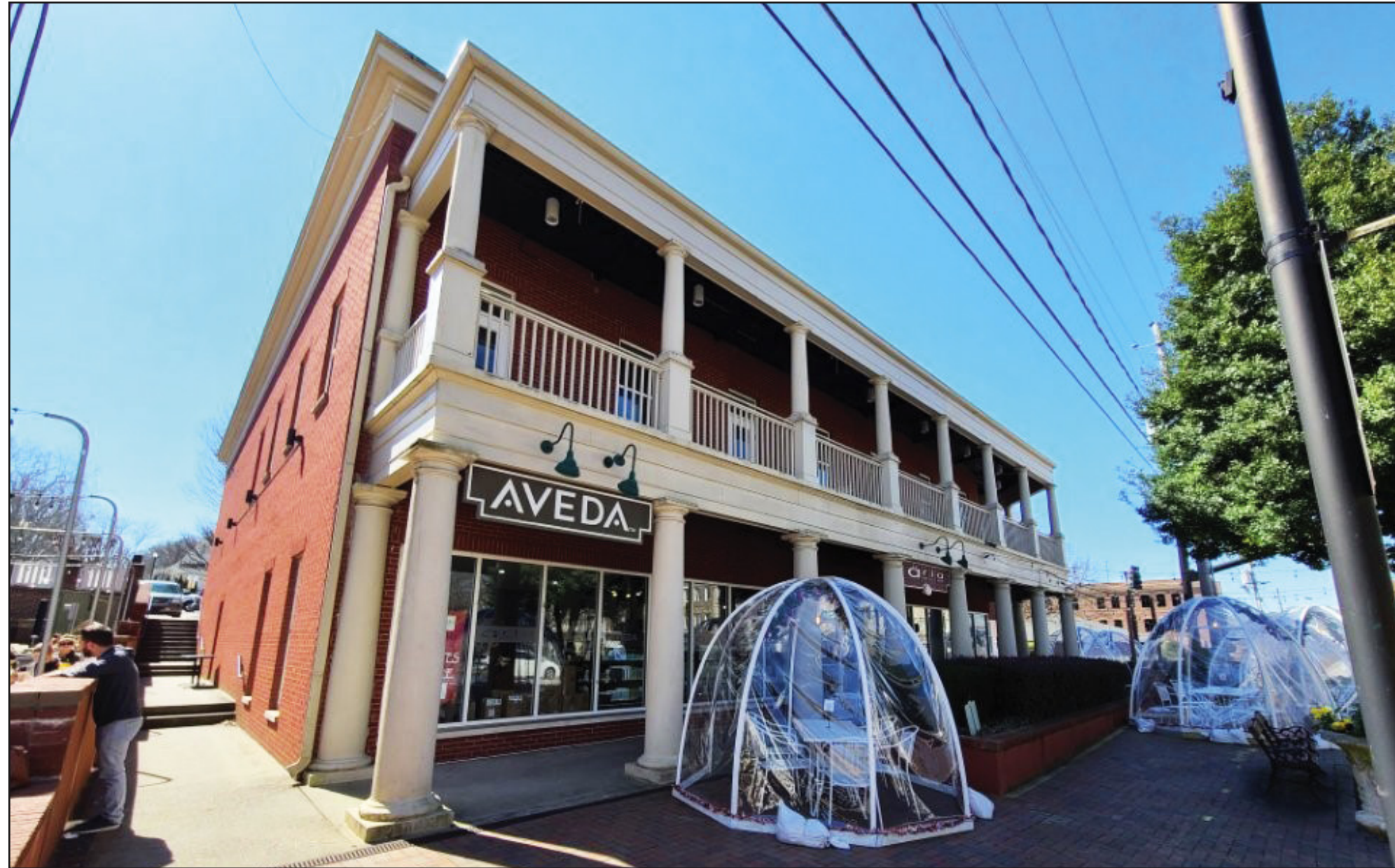
EXISTING BUILDING FACADE
