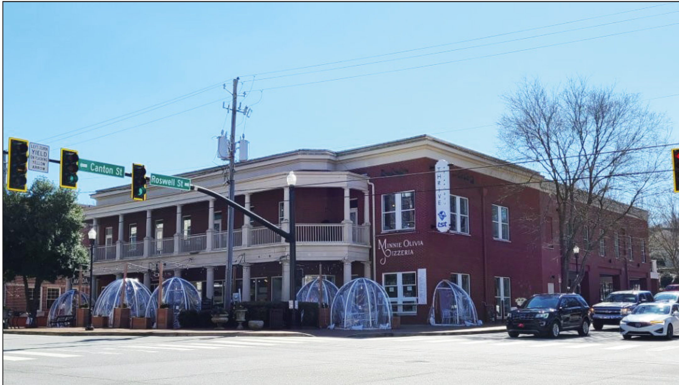
EXISTING BUILDING FACADE
