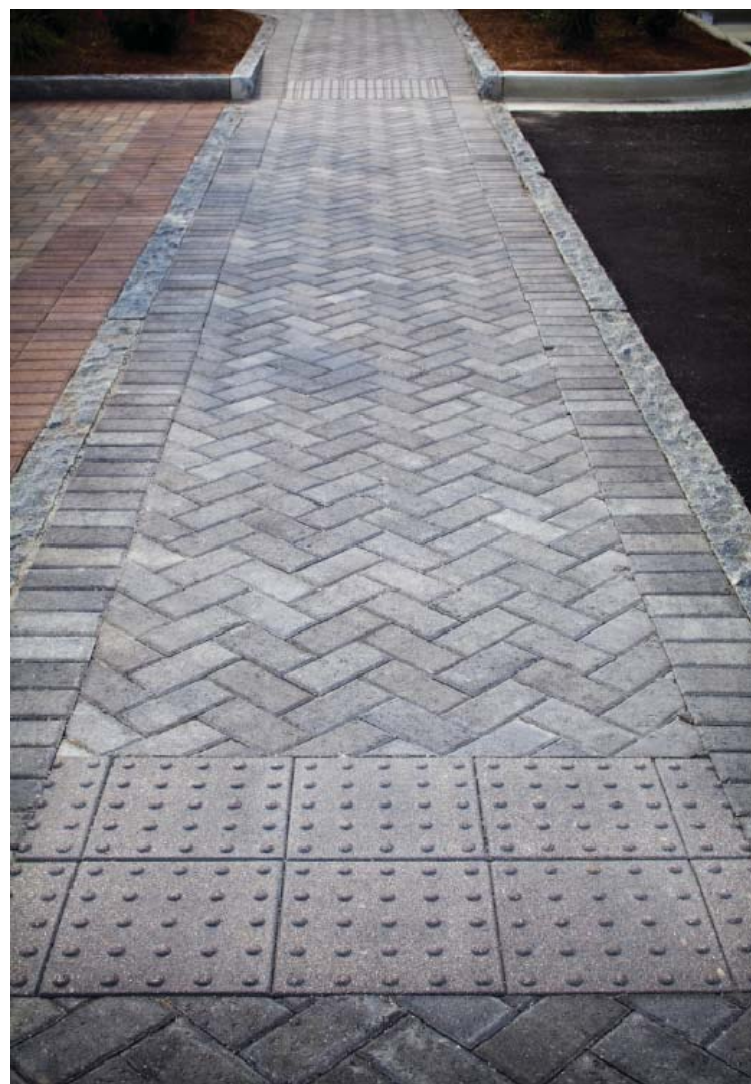
Hanover 'Prest' Brick - Limestone Gray & Charcoal Blend w/Granite Paver Edge
