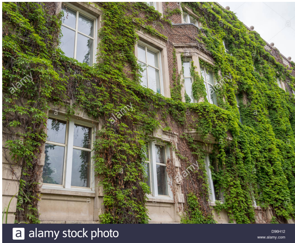
41 Milton Avenue, North Wall
