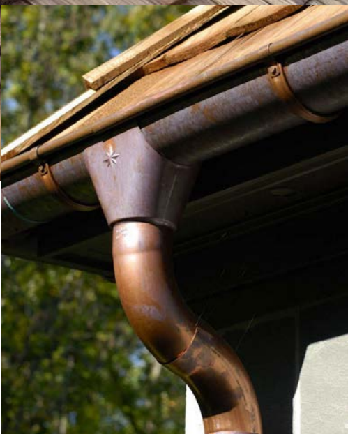
Copper Gutters & Downspouts
