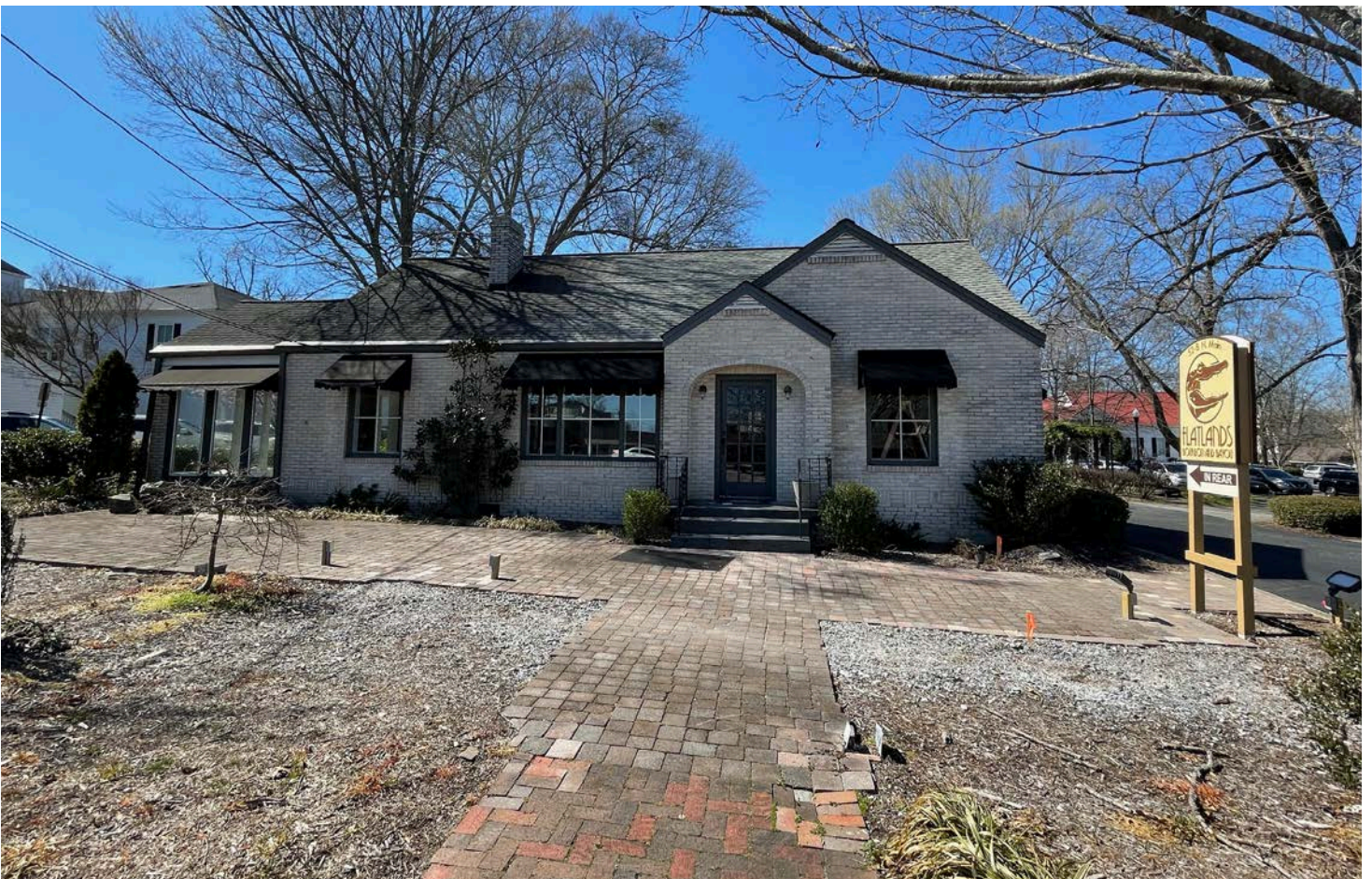
CURRENT VIEW (FROM N. MAIN STREET)
