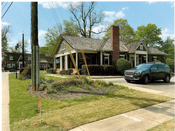
Southeast Façade: Utility pole and guide wires are unattractive and create a hazard in the nearby pedestrian walk paths. Design solution includes creating a neatly low hedged surround to clean edges of awkward utilities with interior of soft colorful blooming plants.
