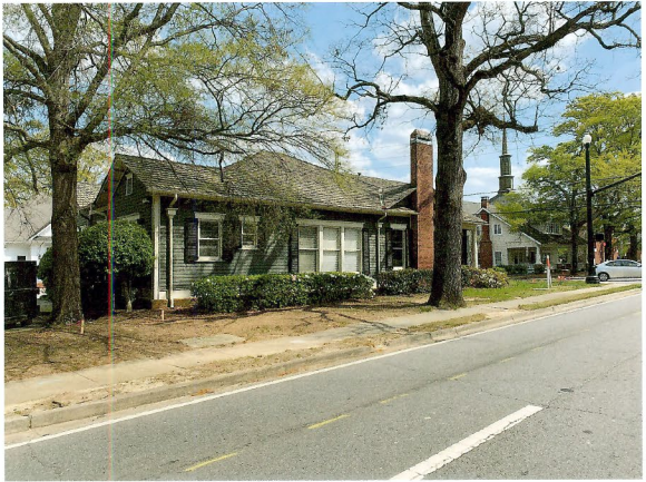
West Facing Façade: Foundation Shrubs are dated and overwhelming the Buildings' Architecture and scale. Solution includes installing a southern pallet of colorful appropriated scaled plantings. Note: This side of the property will need to be phased with slated DOT project along Mainstreet as the ROW encroaches closely to the foundation. Some landscape field review may be necessary once complete to provide best possible landscape solution.
