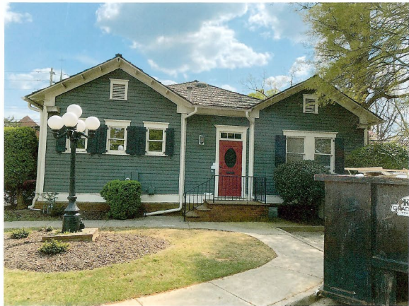
Northside Façade: Smaller bed areas at the foundation of the building lack impact and Air conditioner units lack room for landscape softening. Proposed plan includes installing appropriate foundation planting and recommended fence screen to minimize view of AC units.
