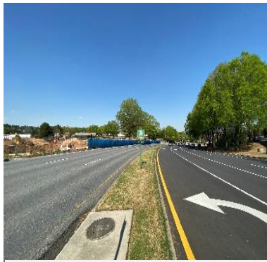
Potential bioswale location
