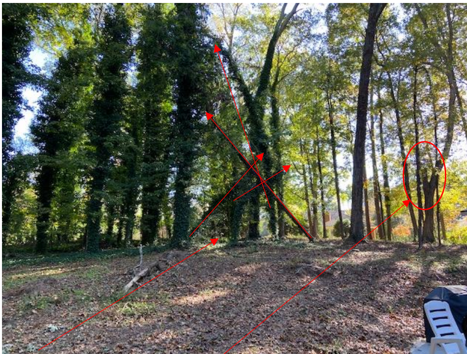
Leaning or failed trees. Previous failure.
