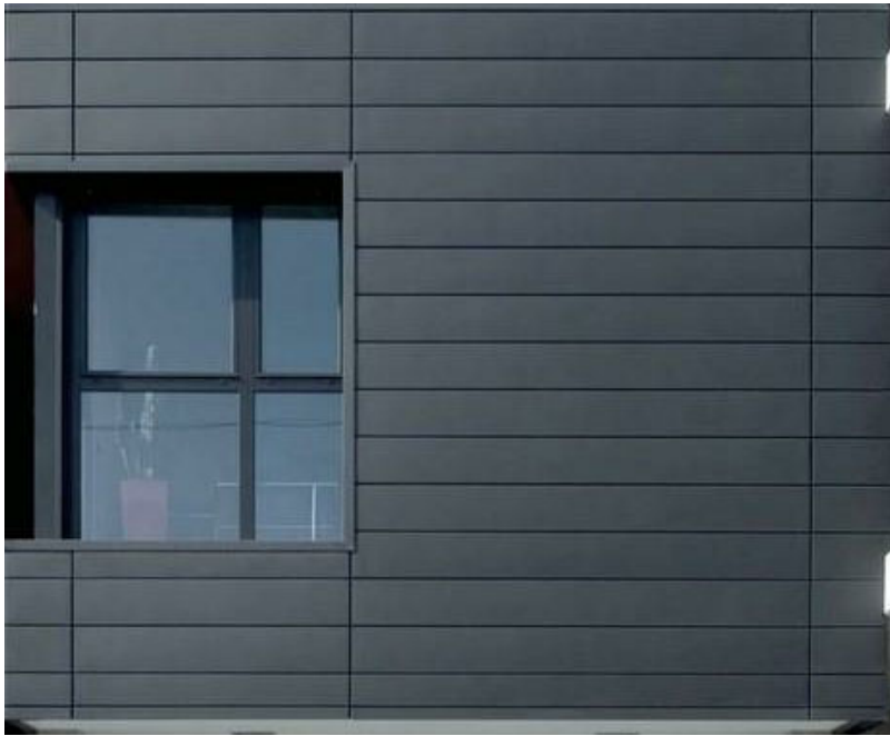
RETAIL/STORAGE SIDING - FIBER-CEMENT PANELS
