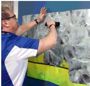
FIGURE 14 Squeegeeing Exposed Adhesive for Self Hinge
