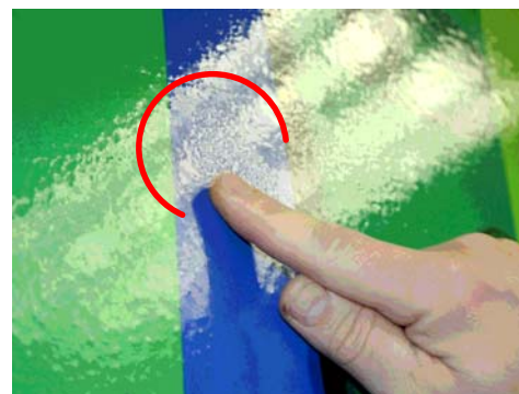
FIGURE 19 Check for Full Adhesive Contact with Wall
