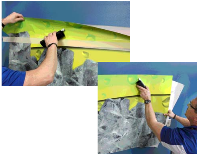
FIGURE 17 Keep Tension on the Unapplied Film
