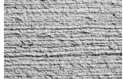
CMU/Concrete Block, Painted/Unpainted Medium Unsmooth Texture Use Textured Surface Film
