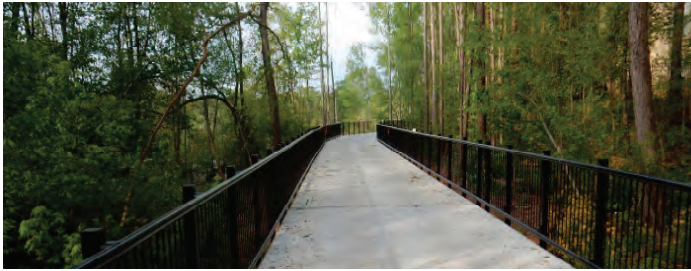
Figure 3. Atkins provided construction management services for the Big Creek Greenway in Alpharetta.
