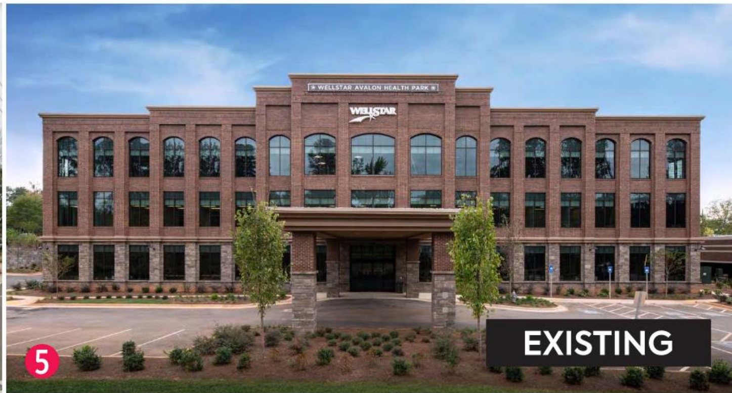
Rear/North Elevation Wall Signage (Existing)
