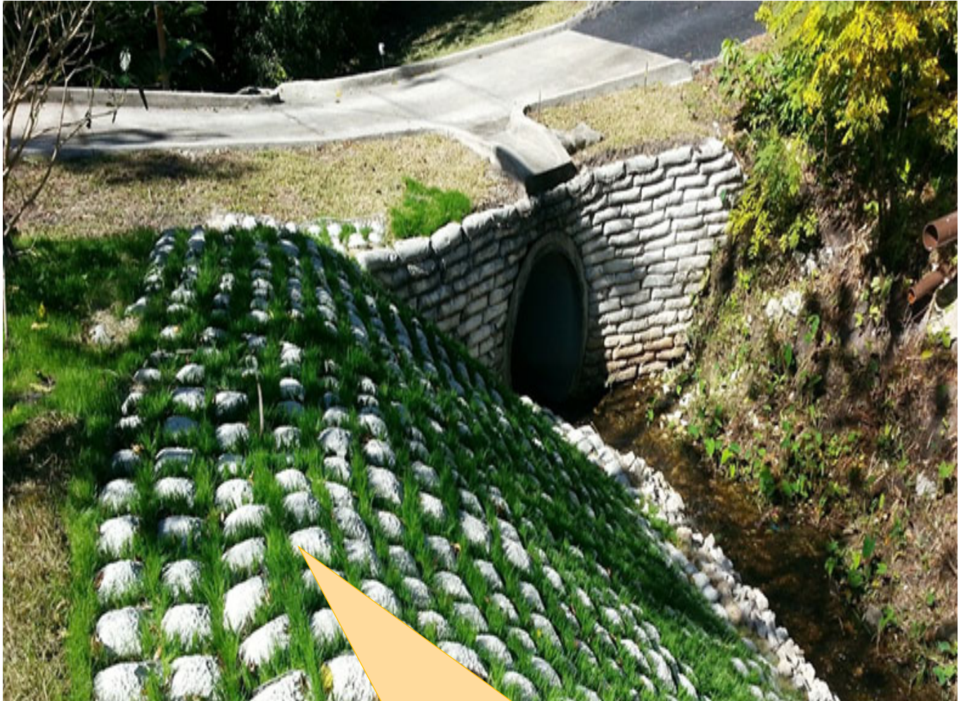
Revetment matting installed on streambank slope with perennial grasses planted in voids.
