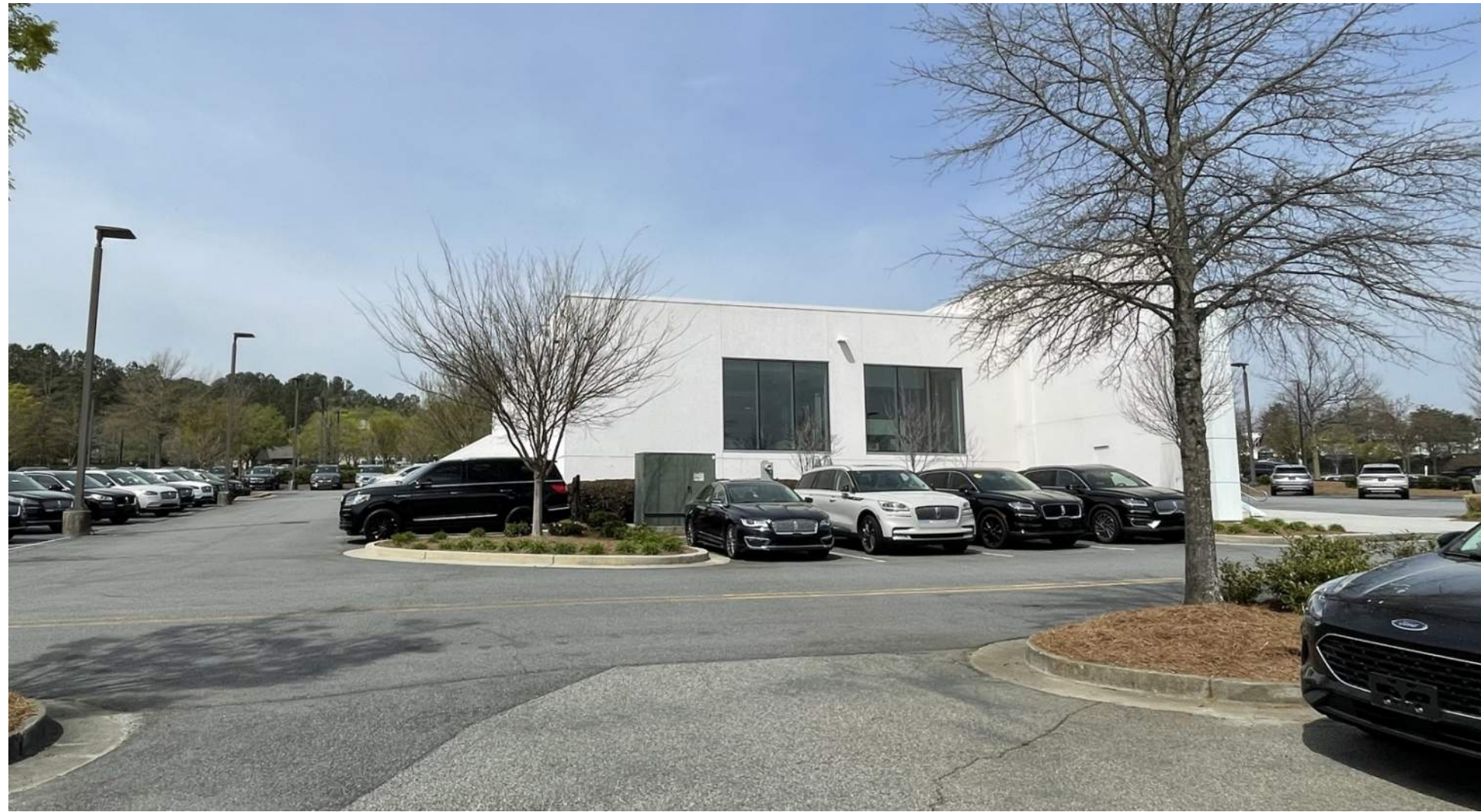
EXISTING PICTURE #1 - EAST ELEVATION
