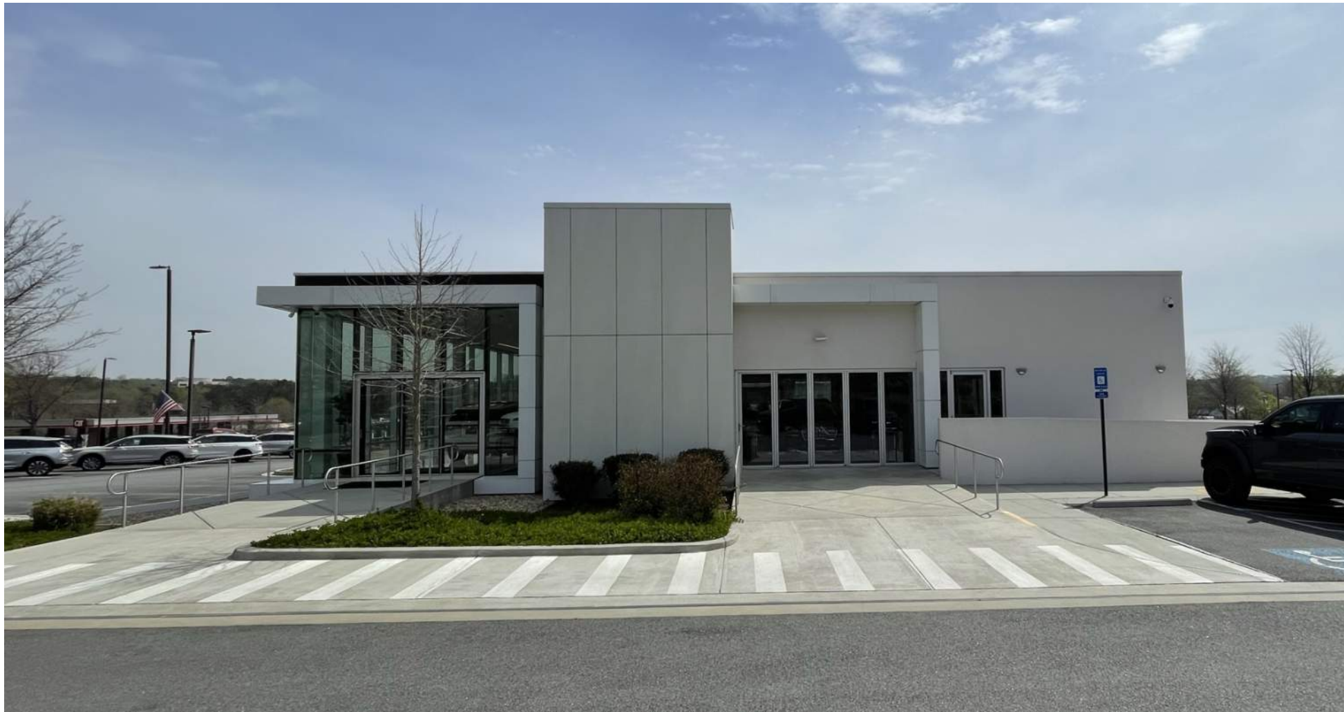
EXISTING PICTURE #3 - WEST ELEVATION
